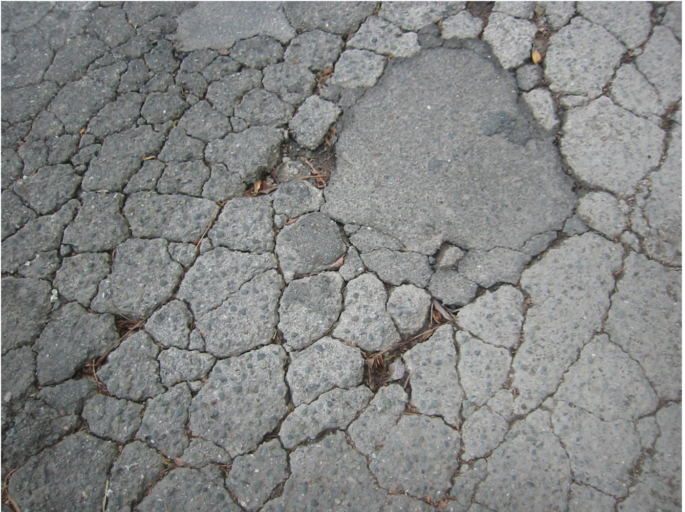
Fig. 8: Closeup of poor pavement condition immediately in the access point on street
