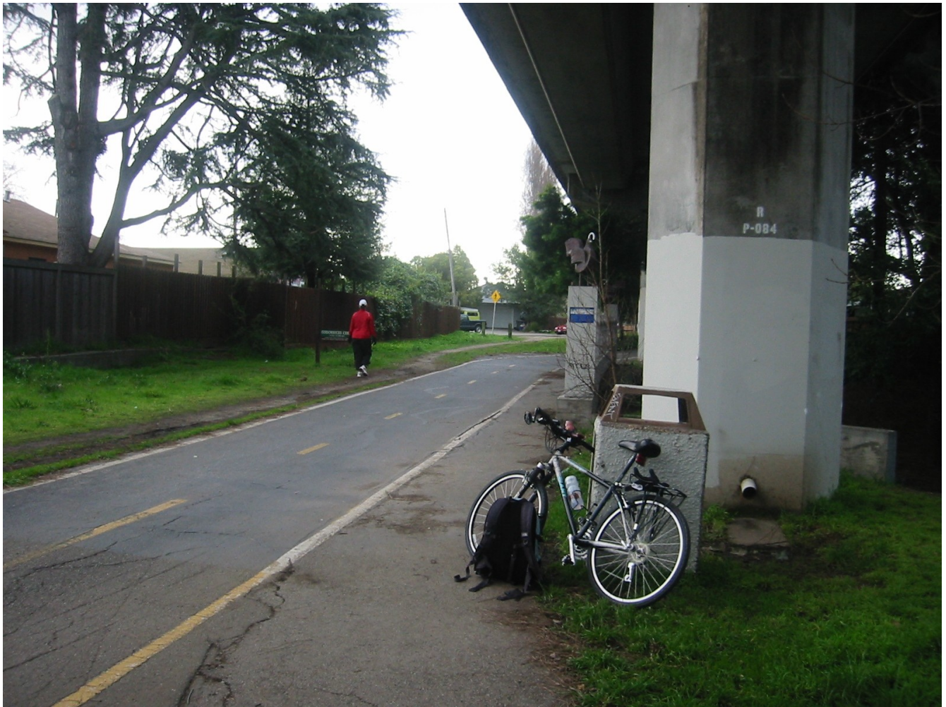
Fig. 12: shared bike/ped path (southwest bound) merging with bike path; peds are forced to the narrow strip on the right, which then ends narrows and ends abruptly in the middle of the creek overcrossing. Suggestion for the eventual reconfig: the path can maybe veer to the left a bit at this point to give those merging from the right some room?
